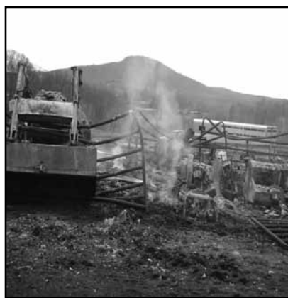
The remains of the Bauer's barn.
