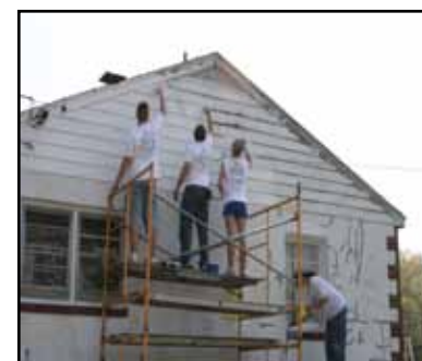
Poolesville Rebuilding Together has a project planned for later in April.
