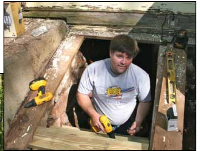
Eddie Schwartzbeck replaces a defective stairway to basement.
