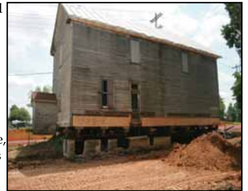
The Old Darby Store in Beallsville is about to move twenty-seven feet.
