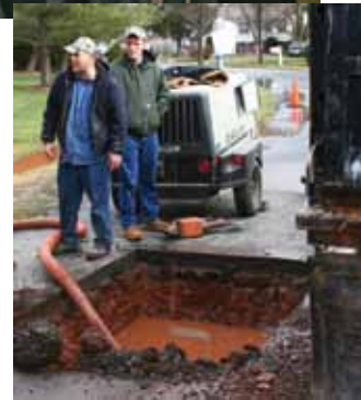
A water line broke, but this team of hard working town employees has done it all before.
