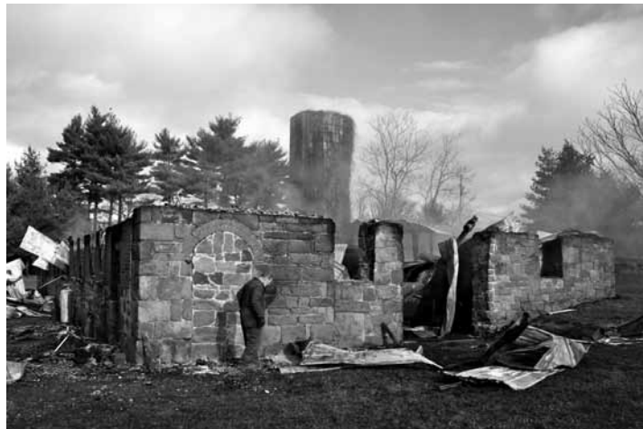
A historic barn at Spates Farm on Westerly Road was destroyed by fire.
