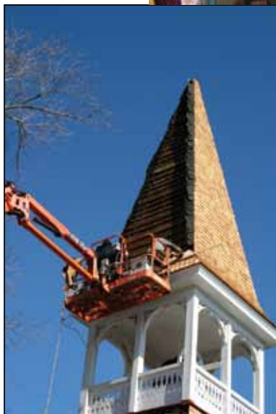
The renovation of the historic St. Peter's steeple is nearly complete and awaits the placement of the cross.
