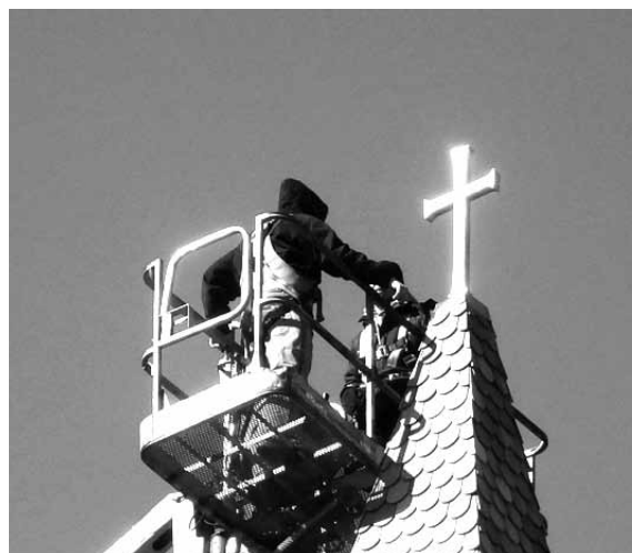
Roofing contractors complete the installation of the new cross at St. Peter’s.
