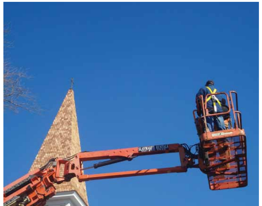
A strapped-in Ted Wroth rides up to inspect the steeple and new cross at St. Peter's.
