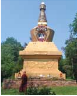
Closed for renovations? The details are in Local News on page 3.
