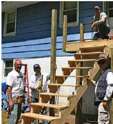
Team Captain Jim Burton (left) supervises a Rebuilding Together project.
