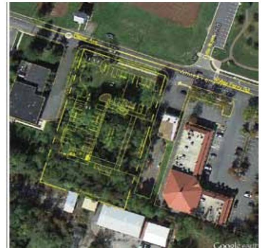
The future site of the Dollar General Store on Fisher Avenue.
