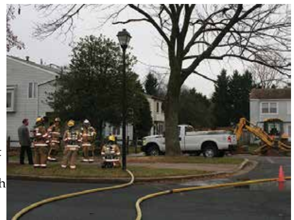
Town Manager Wade Yost and firefighters at the site of a recent gas leak.
