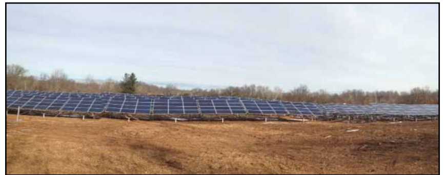
This partial view of the new solar panels in Poolesville is the front section of an array consisting of 3,762 panels located on two sections of property totaling 6.6 acres.
