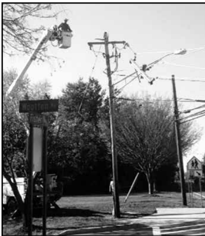
What's left of a transformer dangles dangerously over Fisher Avenue, causing early morning traffic problems in Poolesville.
