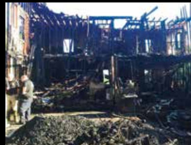
Brian Jamison's home in Point of Rocks was a total loss after a fire started by an electrical problem.
