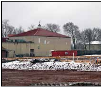
Construction on the new Dollar General store has stopped. Find out why in Business Briefs on page 5.
